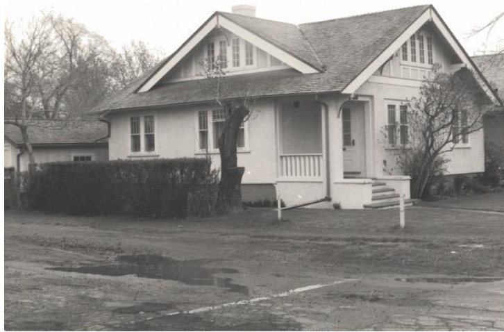
Webb Residence 1984, Alberta Heritage Survey, HS 6123
